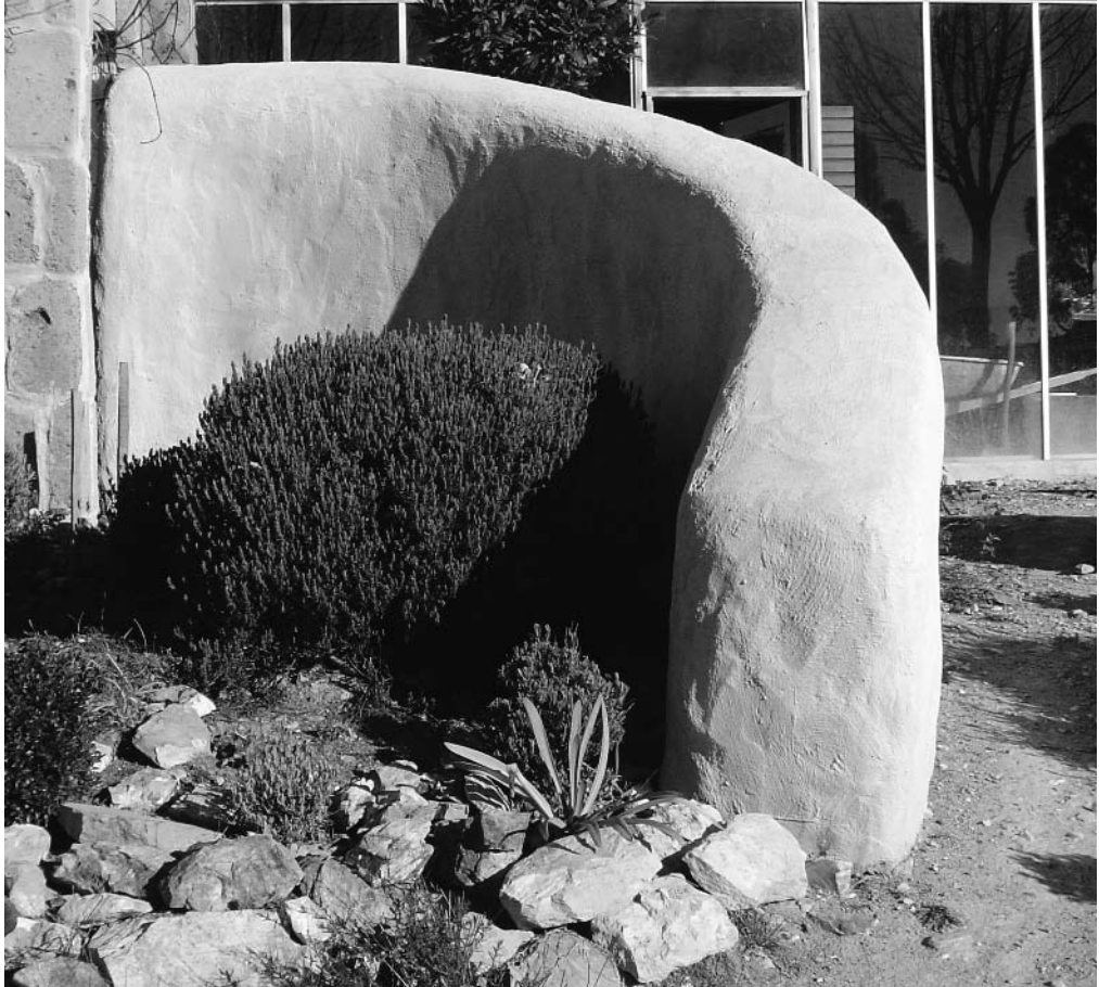
Fig. 28 A curved and tapered wall.
