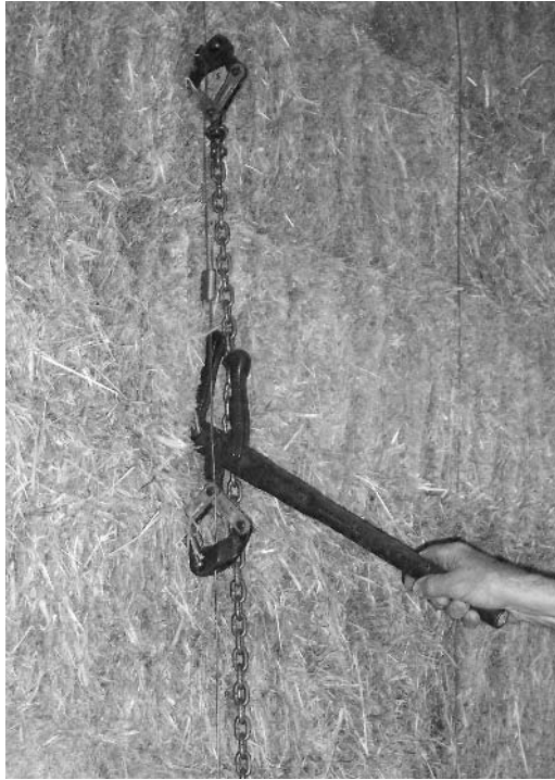
Fig. 11 Using a traditional fence strainer requires a bit of practice.
