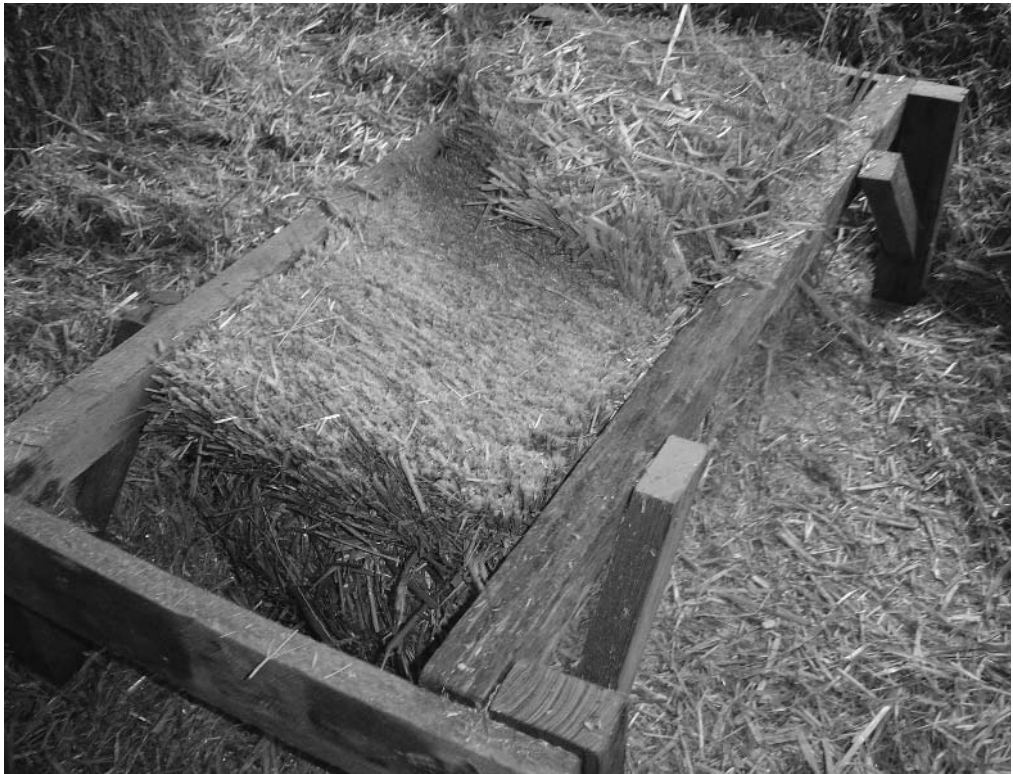
Fig. 21 A bale that has been partially trimmed using a jig: 75 mm is trimmed off one face using a 375 mm-high jig, then the bale is flipped and 75 mm is trimmed off the opposite face using a 300 mm-high jig.
