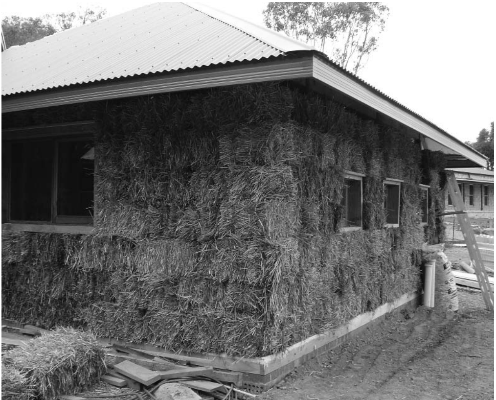
Straw bale house under construction at Jerrabomberra (Queanbeyan, NSW)
